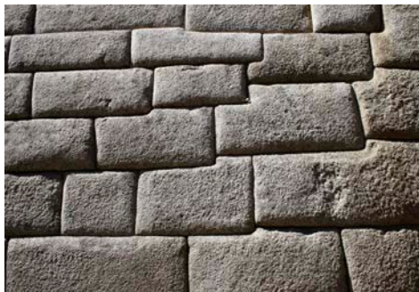
Masonry wall at Machu Picchu.
