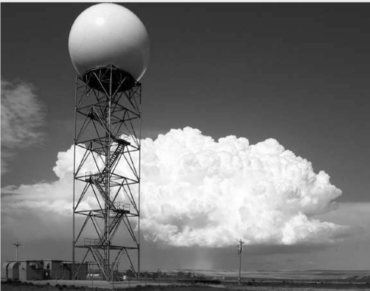
A strong hail producing supercell thunderstorm is depicted in the background with the NEXRAD WSR-88D Doppler weather radar at New Underwood, South Dakota, in the foreground.
