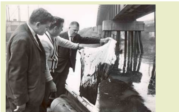
Three Cleveland city councilmen inspect evidence of oil pollution in the Cuyahoga River in September 1964.
