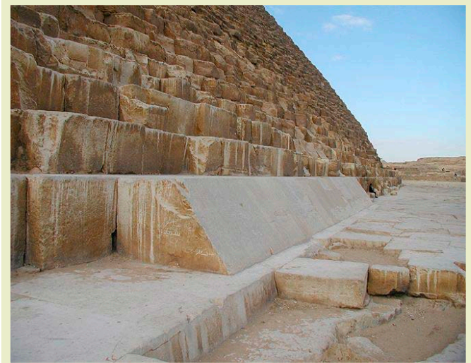
These original Tura Limestone facing stones remain at the base of the north face of the Great Pyramid. They were formed into trapezoidal shapes to give the pyramid its smooth exterior.
