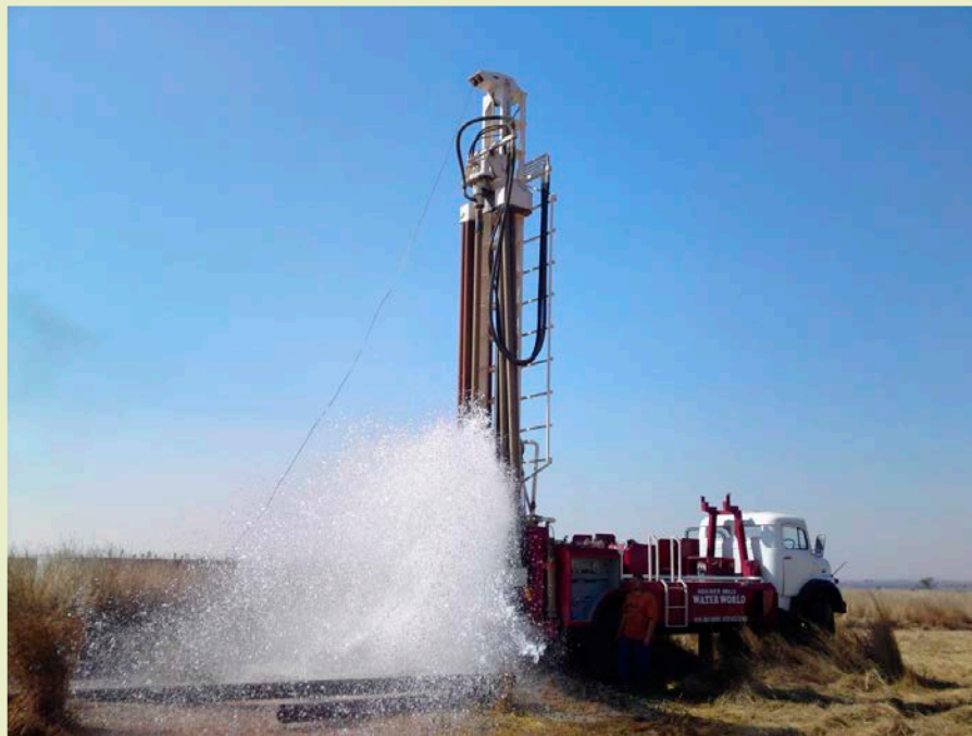
Water flowing from a newly drilled well.
